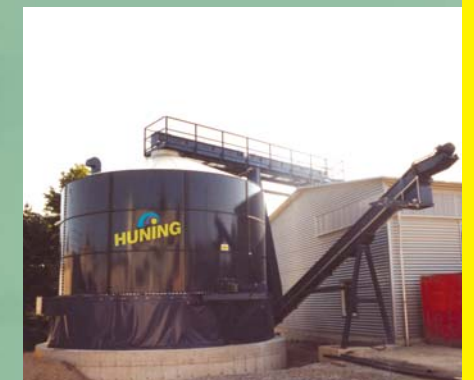
Sewage sludge silo 250 m 3 with screw conveyor; enamelled silo
