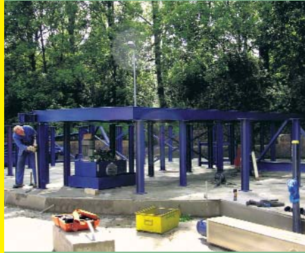
Silo platform designed as a heavy steel sub-structure in bolted construction
